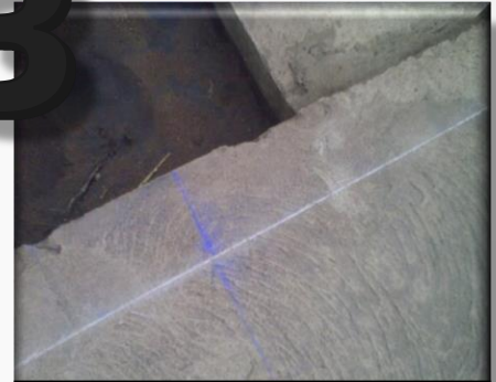
Demarcation on Slab
