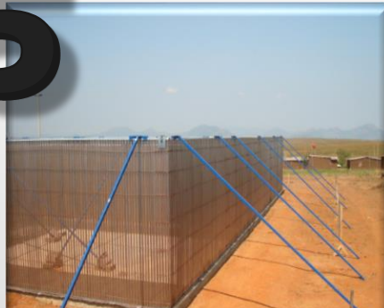
Erection of wall panels
