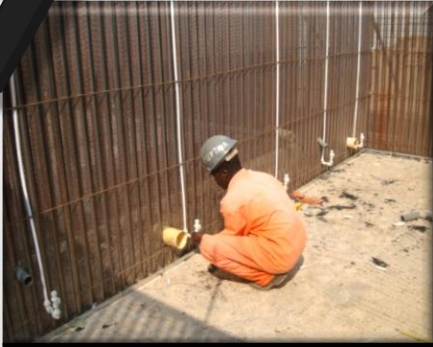
Fitment of in-wall plumbing services
