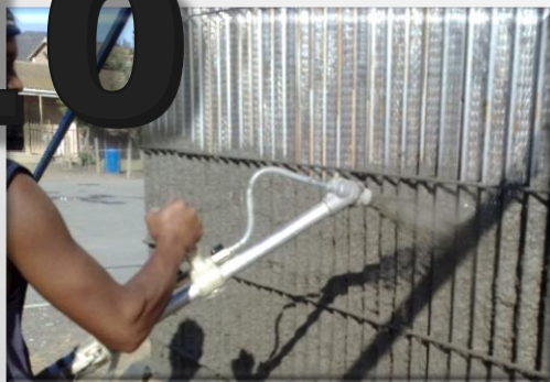
Applying mortar to walls mechanically
