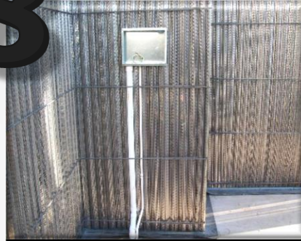
Fitment of in-wall electrical services
