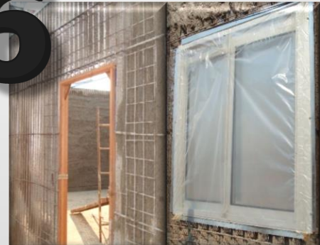
Fitment of door and window frames
