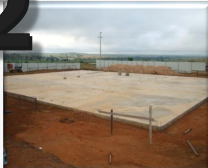
Casting of Raft Foundation
