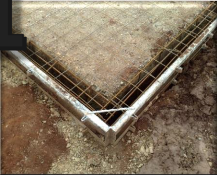
Preparation of Raft Foundation
