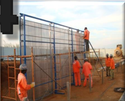
Assembling Wall Panels
