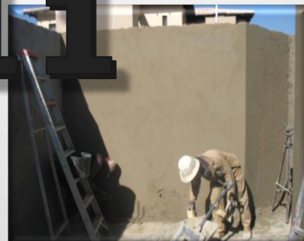
Plaster finish to mortared walls
