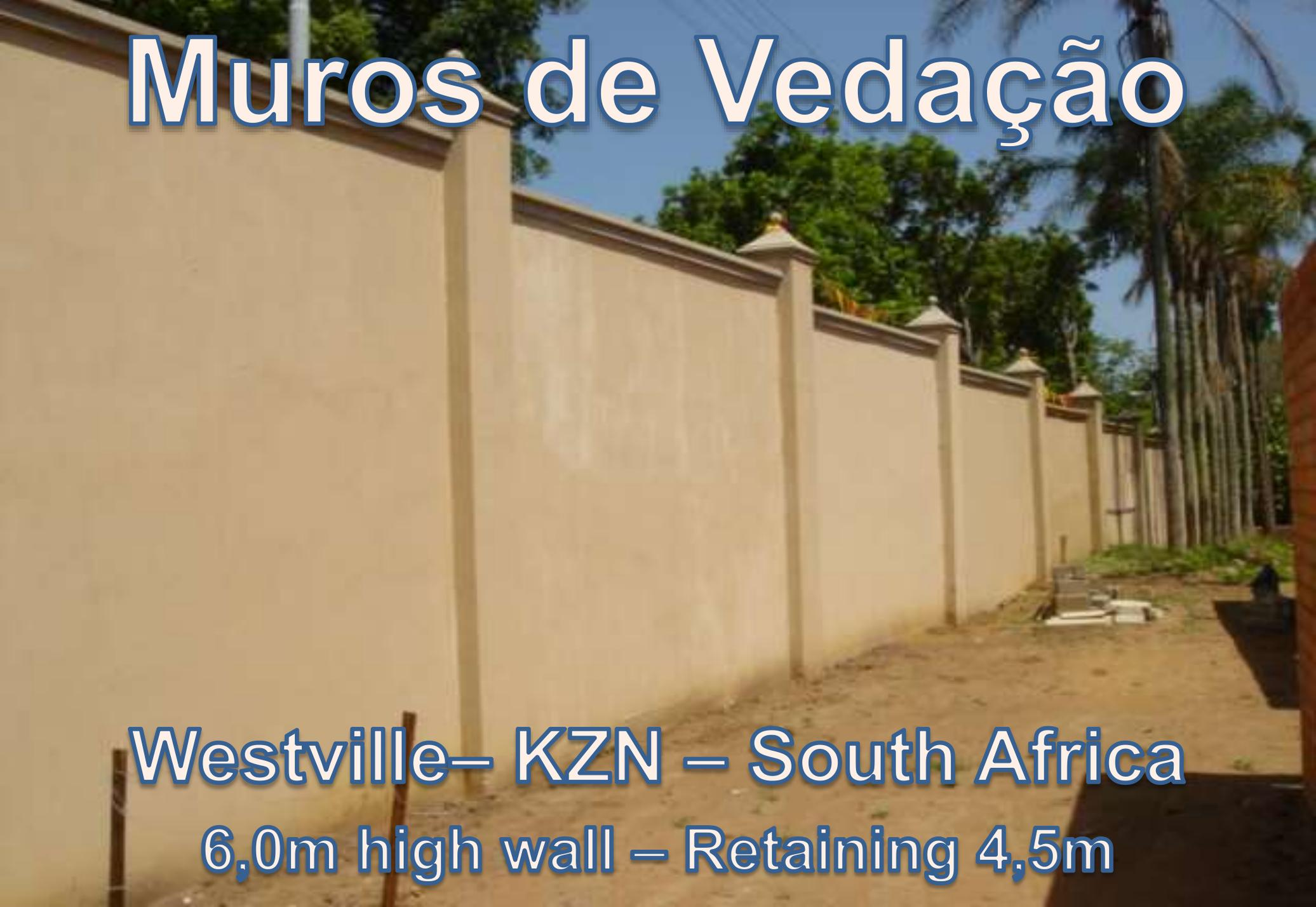
A long, light-colored concrete retaining wall with decorative pillars, set against a background of trees and a clear sky. The wall is built on a dirt embankment and features a series of vertical pillars with decorative caps. The wall is 6.0m high and retains a 4.5m wide area.
